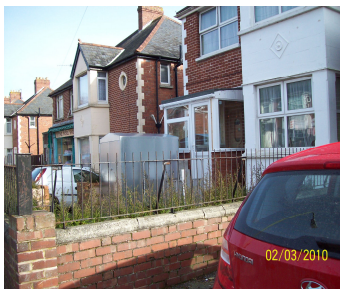
Metal structure in front garden
